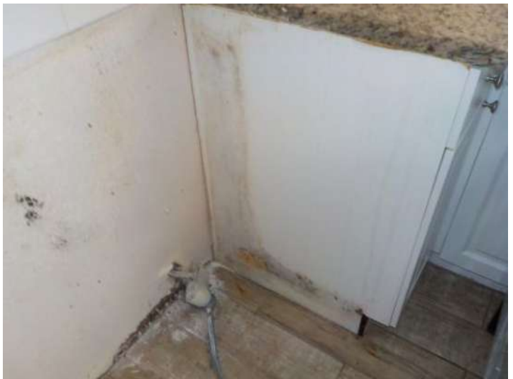
Recommend remove and repair if possible lower kitchen cabinets.
