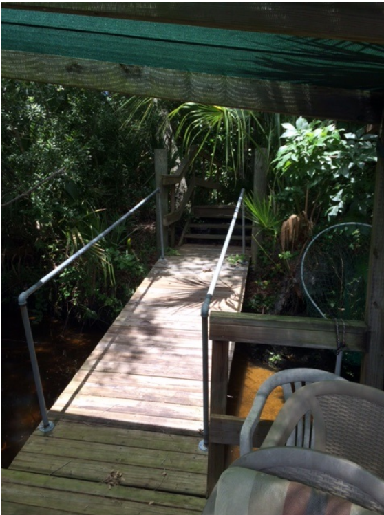
View of dock on Hall/Friday Property
