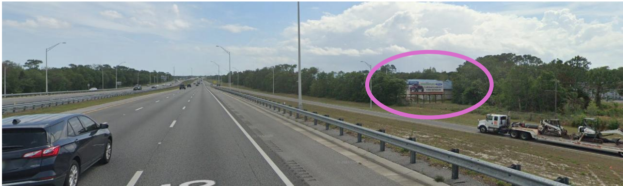
Figure 2. Billboard along I-95 southbound, at the Dunlawton Avenue/Taylor Road interchange proposed to be rebuilt with a digital sign face.
