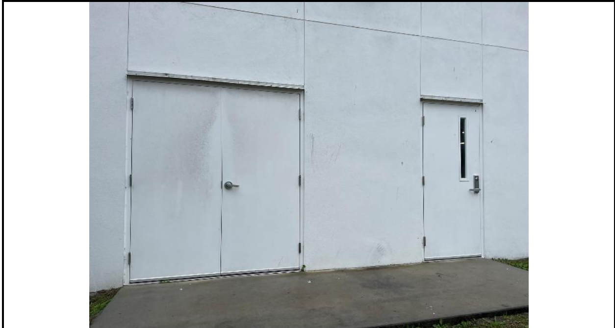
Photo 9: Fenestrations include aluminum-framed fixed window systems and aluminum framed storefronts and entrances as well as hollow core metal doors situated in metal framing with and without glass lites at service/mechanical room entrances.
