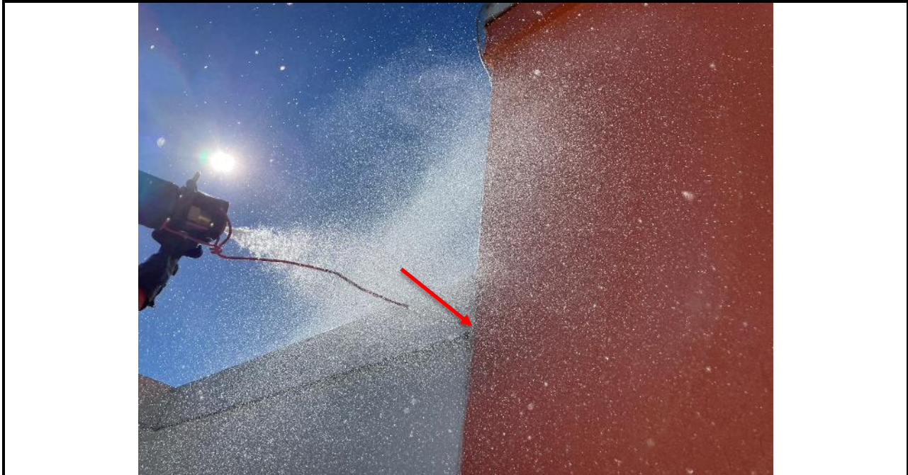
Photo 105: Test location #1 - water was applied along the voids in expansion/control sealant joints (along the stair tower and between the stair tower and elevator penthouse).
