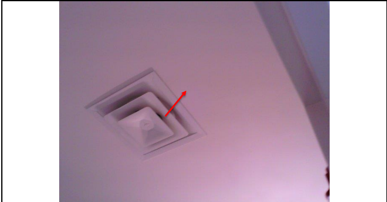
Photo 95: Moisture measurement readings and infrared images were taken prior to commencing moisture infiltration testing typical within equilibrium moisture content (EMC) tolerances correlating to dry or elevated interior finishes/construction components.
