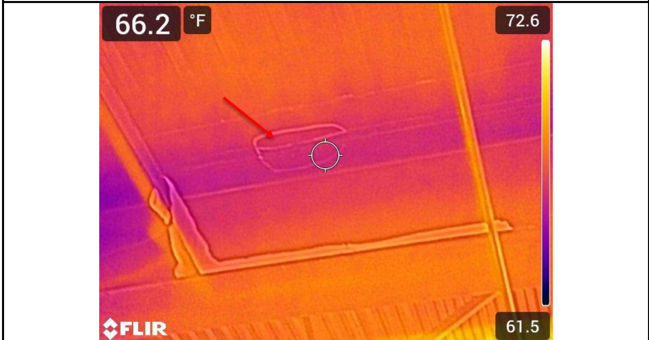
Photo 96: Moisture measurement readings and infrared images were taken prior to commencing moisture infiltration testing typical within equilibrium moisture content (EMC) tolerances correlating to dry or elevated interior finishes/construction components.
