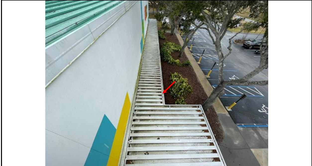
Photo 23: The front (north) elevation consists of a canopy covering the concrete flatwork constructed of metal roof panels supported by steel framing with drainage achieved to gutter and downspout systems discharging water onto the grade below.
