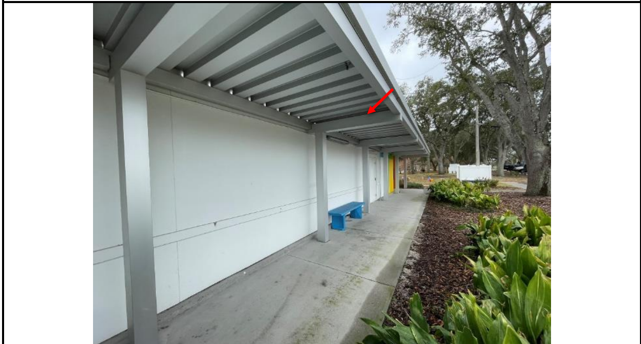
Photo 24: The front (north) elevation consists of a canopy covering the concrete flatwork constructed of metal roof panels supported by steel framing with drainage achieved to gutter and downspout systems discharging water onto the grade below.
