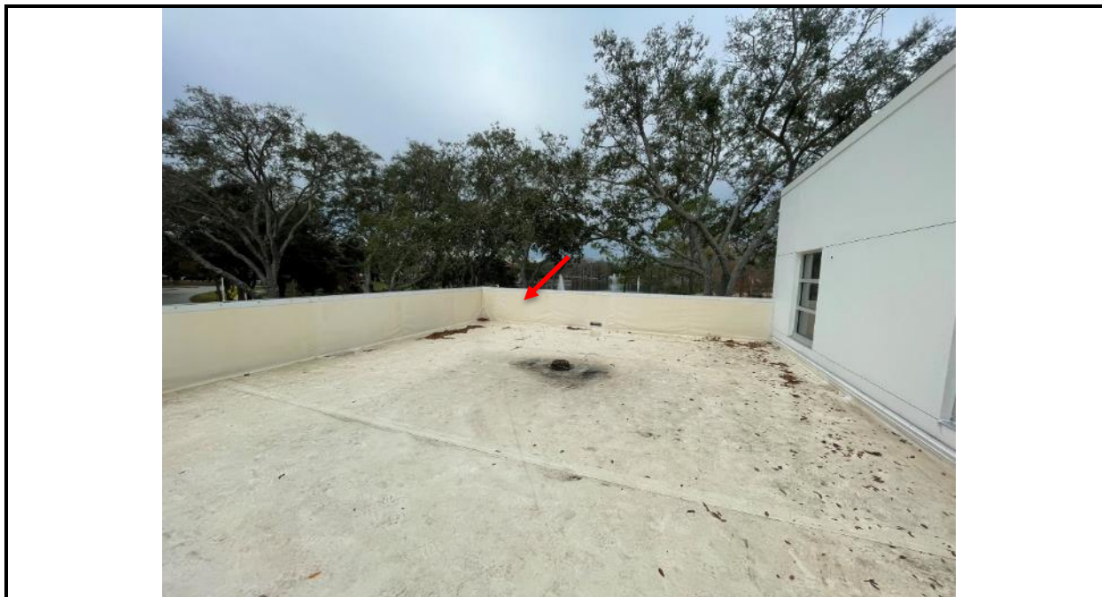
Photo 21: Parapet walls of varying heights bound the low-sloped single-ply membrane roof areas consisting of membrane overlapping the field and terminating beneath metal coping cap or at metal termination bars with sealant joints at adjacent construction components.
