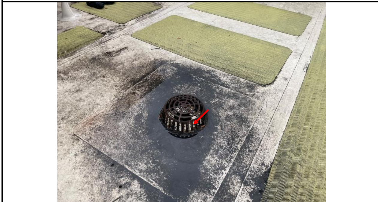
Photo 18: Drainage associated with the remaining roof sections was achieved via sheet flow to primary internal roof drains and emergency through wall scupper systems, ultimately dispersing water into below-grade municipal systems.
