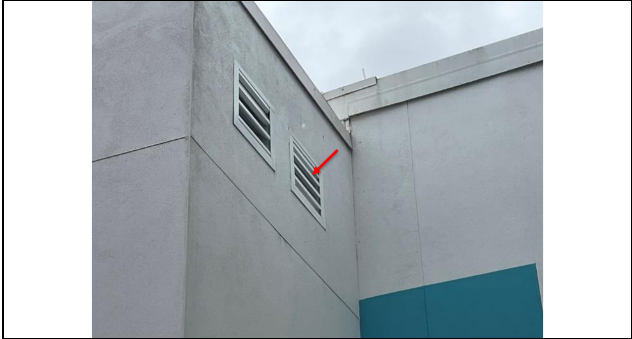
Photo 11: Metal louvers with metal framing are situated throughout building elevations associated with mechanical rooms.
