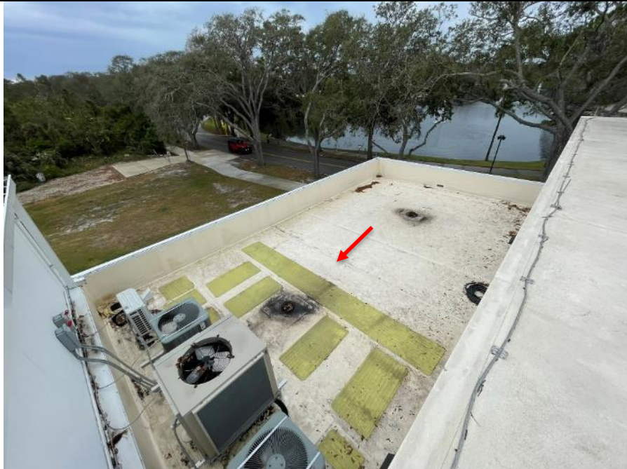
Photo 13: The roof systems associated with the building appeared to consist of a combination of standing seam metal roof panels (over the original construction) and single-ply membrane (TPO or PVC) over the additions.
