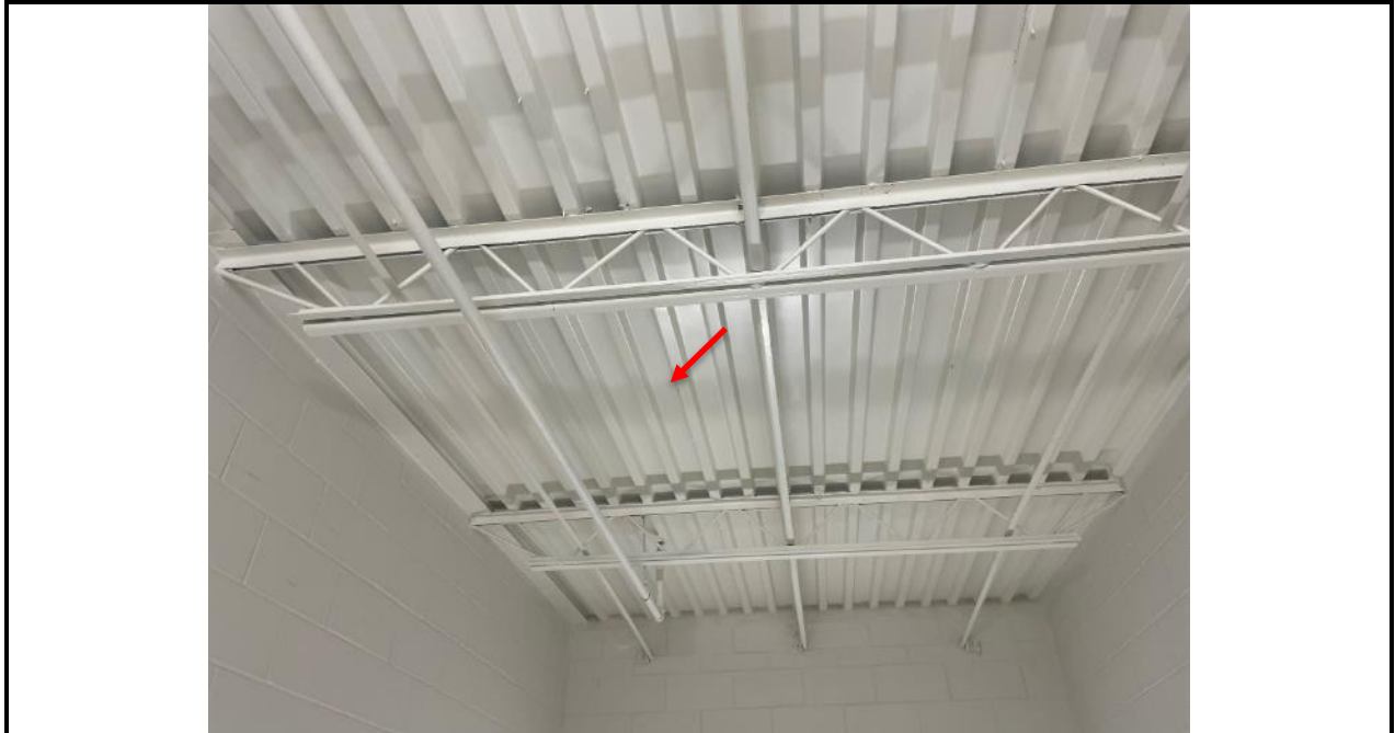
Photo 15: Roof construction appeared to be supported by corrugated steel decking and open web joist/girder systems.
