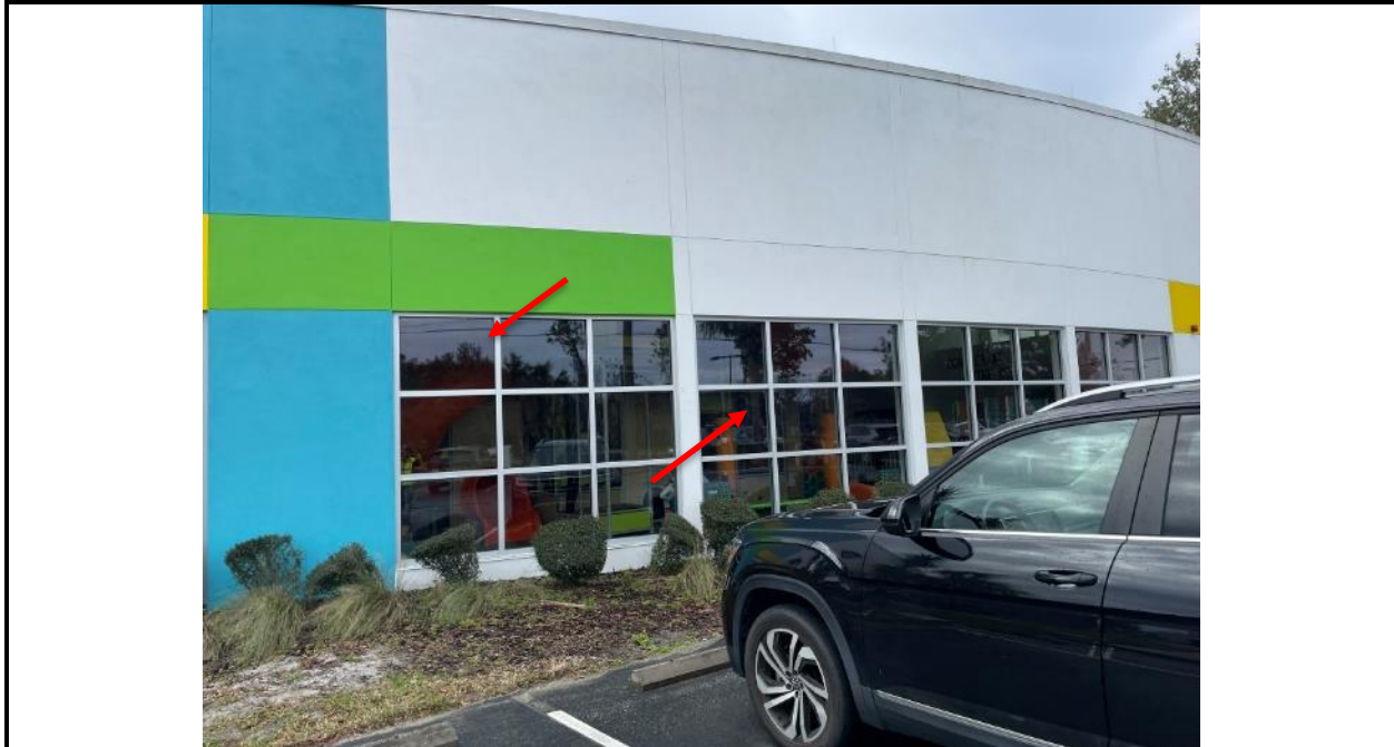
Photo 7: Fenestrations include aluminum-framed fixed window systems and aluminum framed storefronts and entrances as well as hollow core metal doors situated in metal framing with and without glass lites at service/mechanical room entrances.
