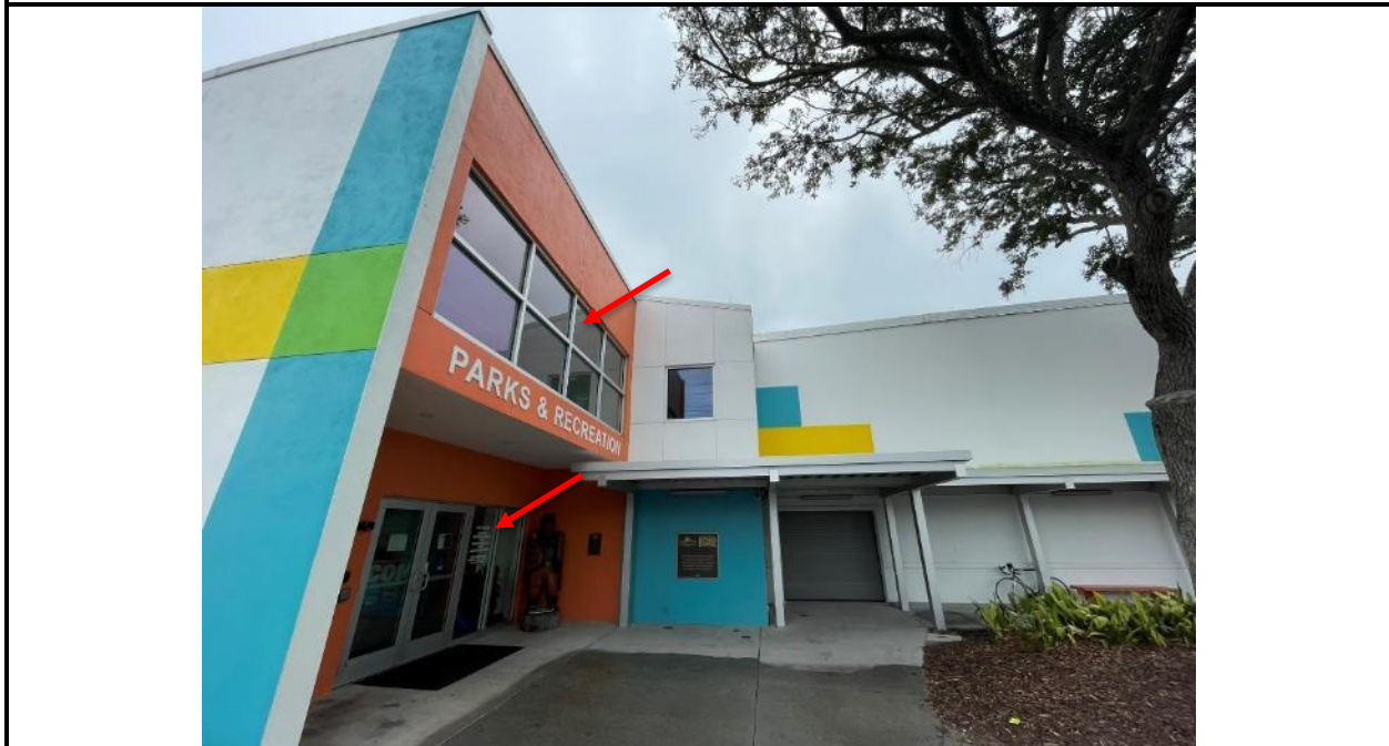
Photo 8: Fenestrations include aluminum-framed fixed window systems and aluminum framed storefronts and entrances as well as hollow core metal doors situated in metal framing with and without glass lites at service/mechanical room entrances.
