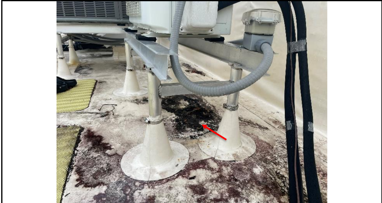
Photo 27: Stained roofing surfaces (membrane).
