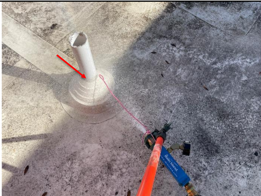
Photo 100: Test location #1 - water was applied along the roof penetrations including roof drain, deteriorated/missing sealant at roof penetrations (VTR) and building component transitions (coping cap to stucco cladding).
