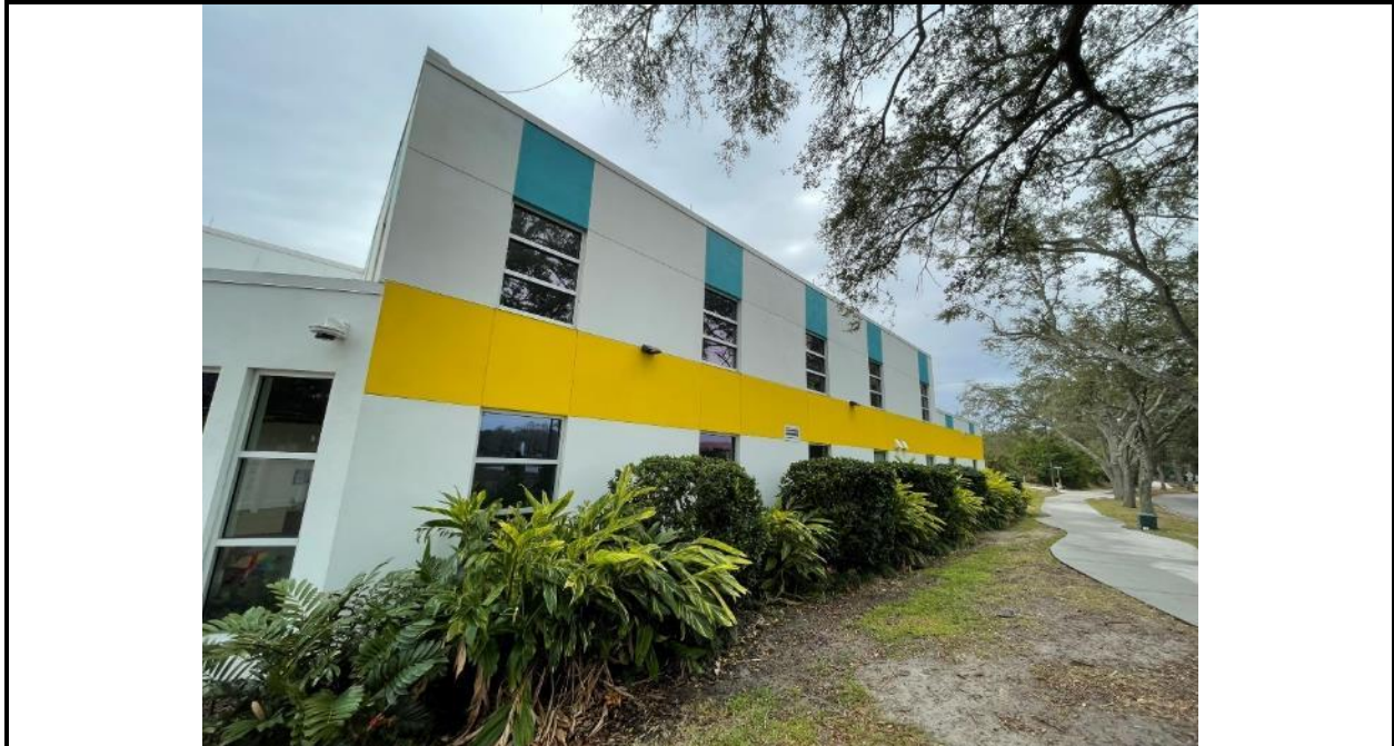
Photo 3: General overview of the Port Orange Recreational Center - East Elevation.
