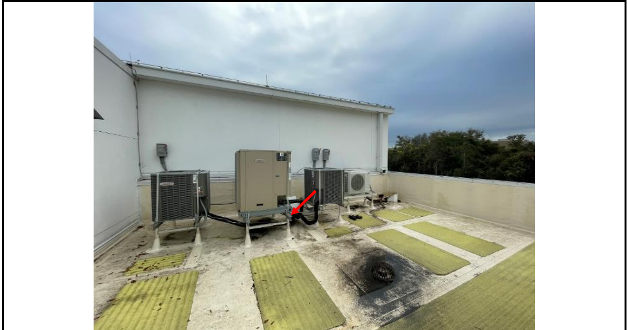
Photo 20: Roof penetrations include HVAC stations, vent through roof (VTR) piping, mechanical equipment curbs, exhaust fan curbs, and lightning protection.
