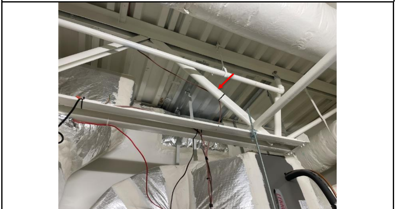
Photo 16: Roof construction appeared to be supported by corrugated steel decking and open web joist/girder systems.
