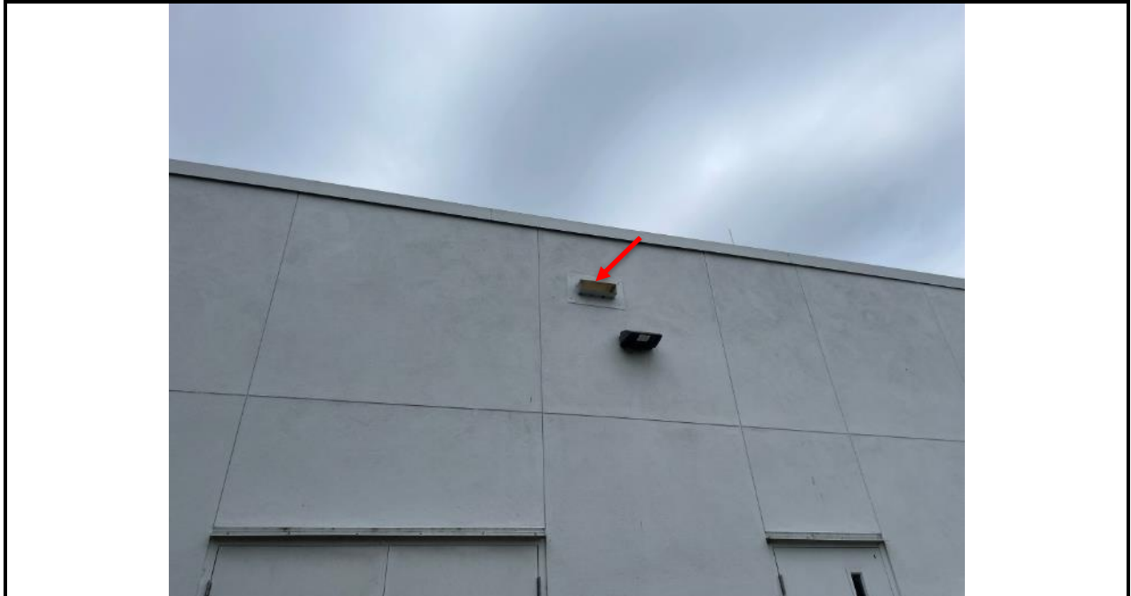
Photo 19: Drainage associated with the remaining roof sections was achieved via sheet flow to primary internal roof drains and emergency through wall scupper systems, ultimately dispersing water into below-grade municipal systems.
