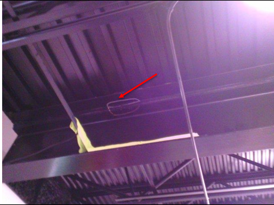
Photo 97: Moisture measurement readings and infrared images were taken prior to commencing moisture infiltration testing typical within equilibrium moisture content (EMC) tolerances correlating to dry or elevated interior finishes/construction components.
