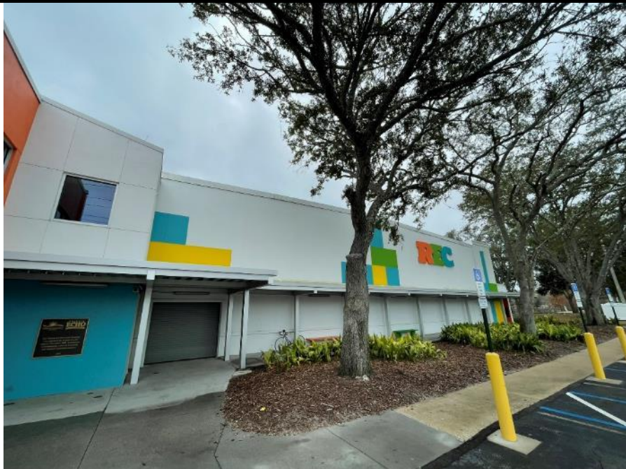
Photo 6: The building’s exterior cladding systems consisted of a combination of Exterior Insulation Finish System (EIFS) with decorative bands (original construction) and direct applied stucco with paint finishes (east and west additions).
