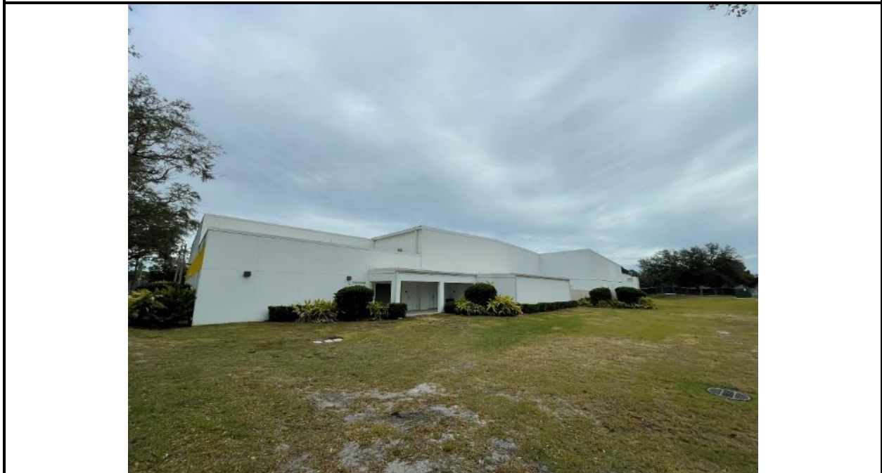
Photo 4: General overview of the Port Orange Recreational Center - South Elevation.
