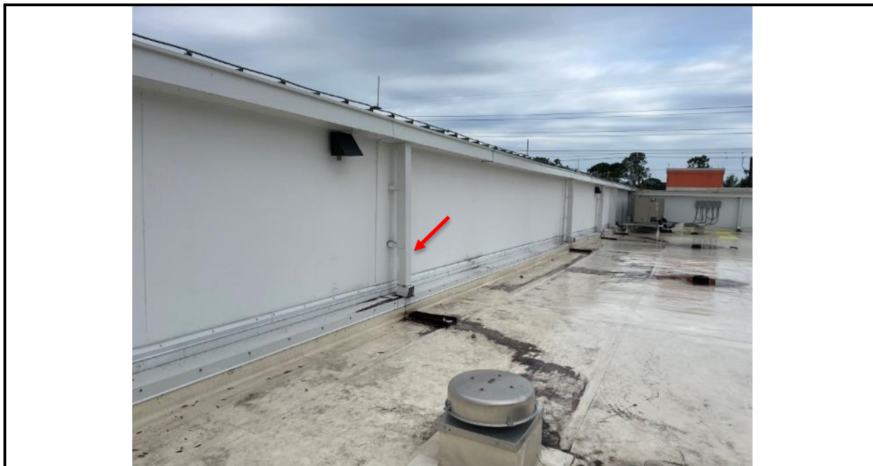
Photo 17: Drainage of upper roof sections was achieved via sheet flow to roof perimeters where water is collected into gutter and downspout systems, ultimately discharging water onto splash block throughout lower roof areas.
