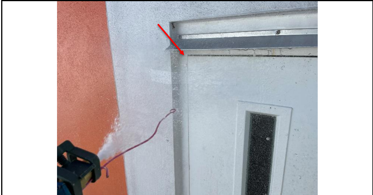
Photo 111: Test location #3 -water was applied along the roof access door perimeters and diverting flashing above the entrance.
