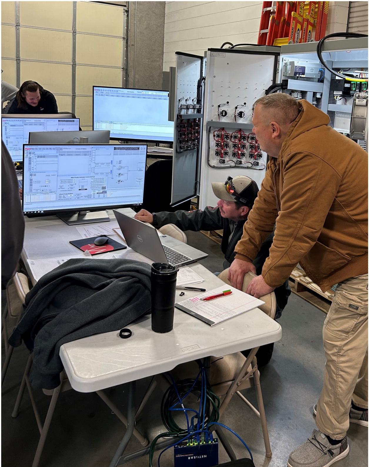
City Staff Inspecting Controls Equipment at Witness Testing
