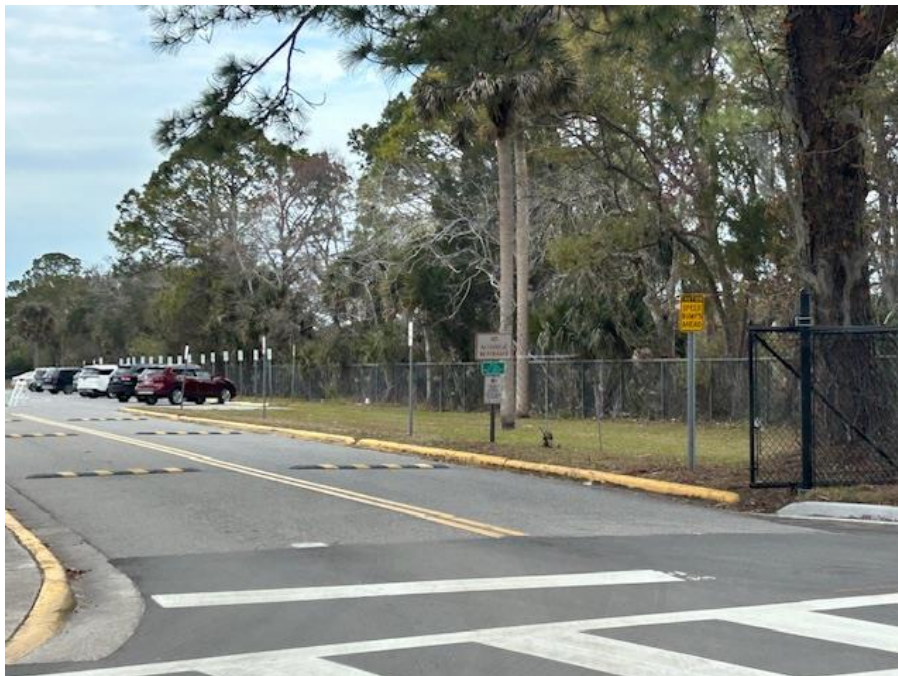
Picture of existing 6-foot chain link fence and existing vegetation buffer adjacent to the subdivision
