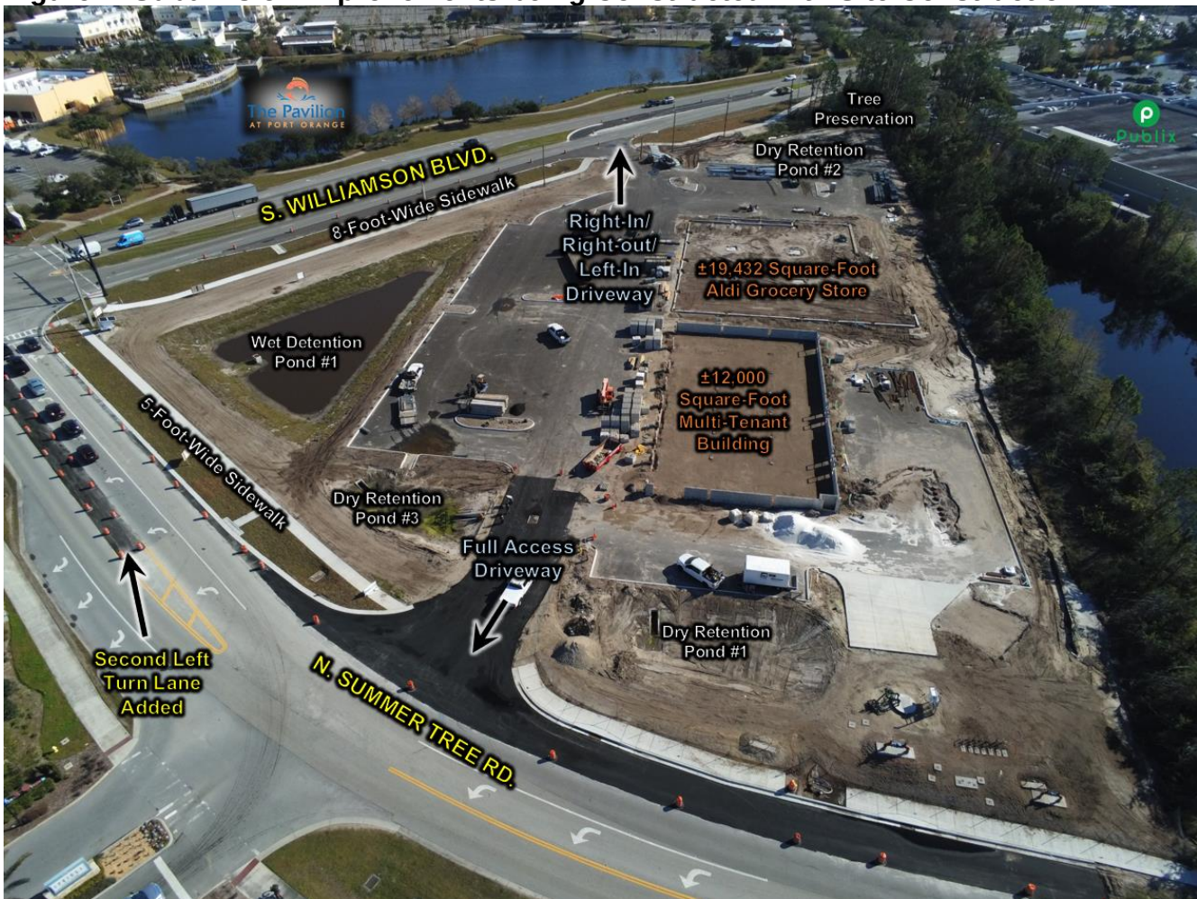
Figure 2. Subdivision Improvements being Constructed with Site Construction
