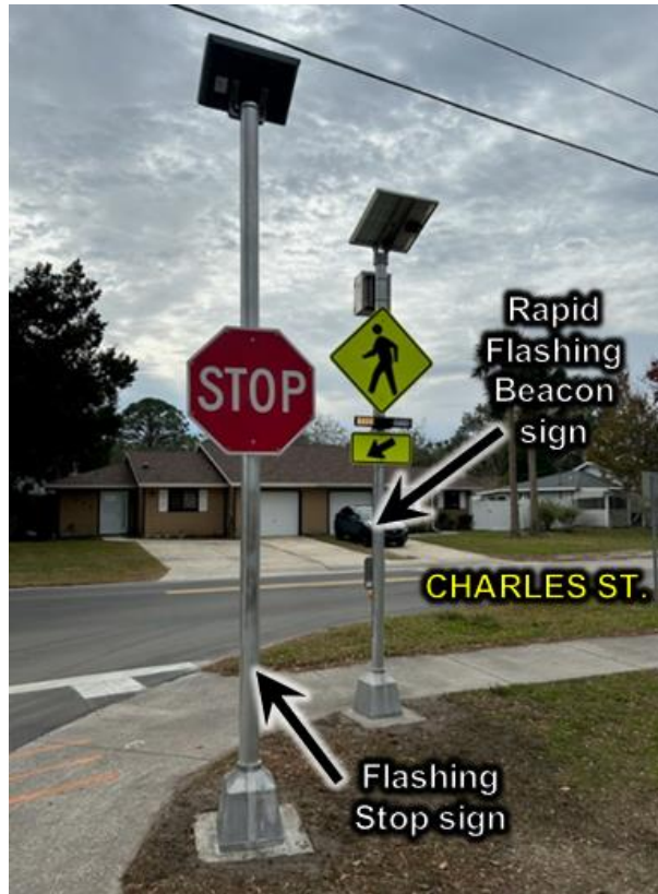
Picture of a Rapid Flashing Beacon sign and Flashing Stop sign installed at Sugar Mill Elementary pick-up/drop-off driveway on Charles Street
