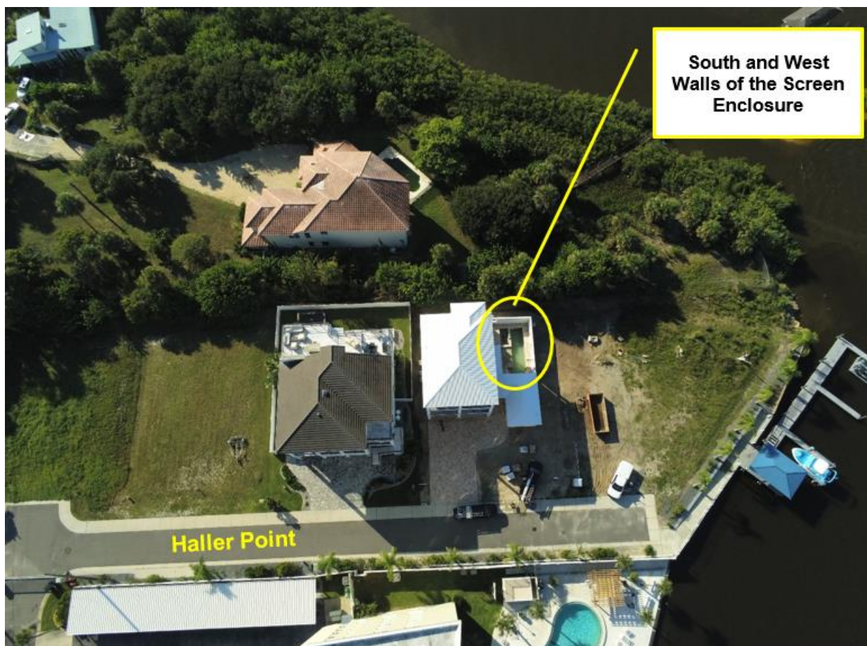
Aerial photo of the Single-Family Home and Screen Enclosure on Lot 4 of the Angler's Cove Subdivision
