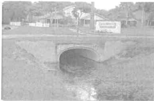
Concrete culvert under Rockledge Lane (standing west of Rockledge Lane, facing east).
