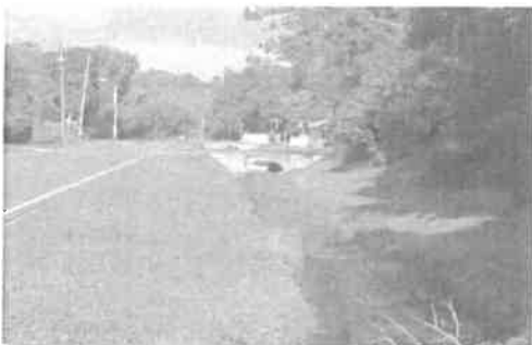
Drainage ditch along Jackson Street (standing west of Rockledge Lane, facing east).
