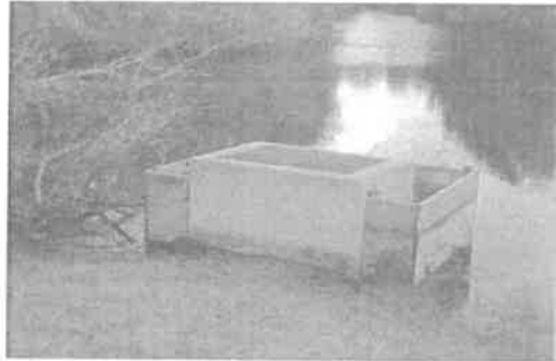
Control structure associated with Woodlake Subdivision (standing near Sanders Road, east of Alder Drive).
