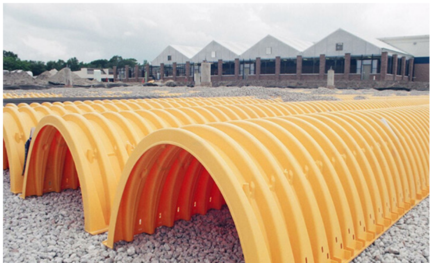
UNDERGROUND STORMWATER CHAMBERS
