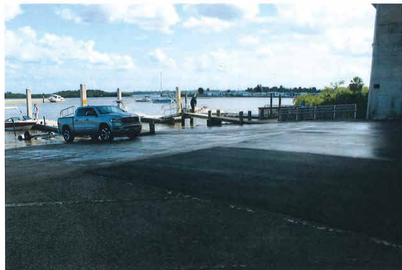
EXISTING BOAT RAMP FACING SOUTH DMC 07/21/2023
