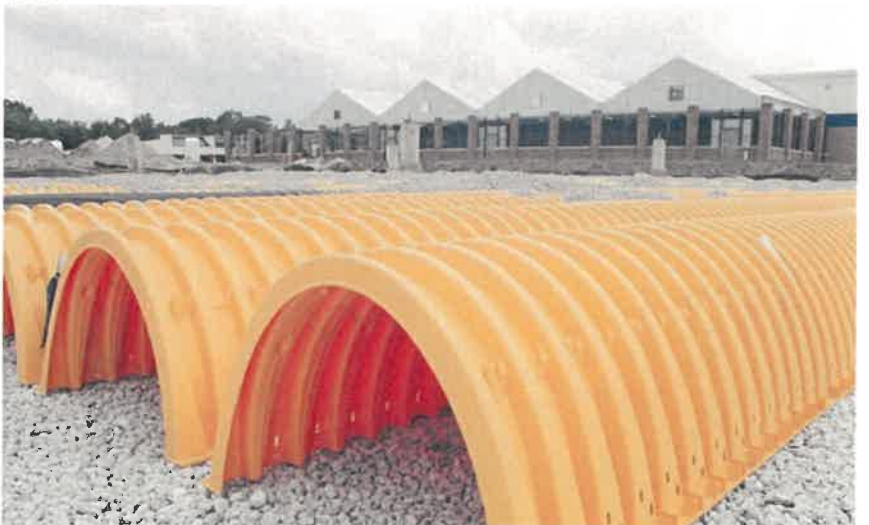
UNDERGROUND STORMWATER CHAMBERS
