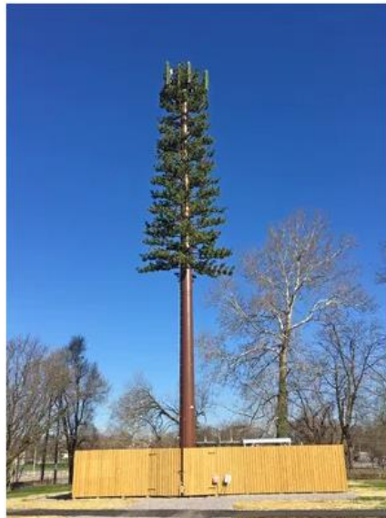
Figure 4. Example of a monopine communications tower
