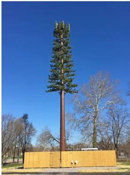
Figure 4. Example of a monopine communications tower
