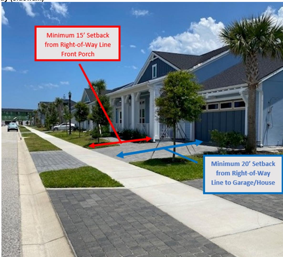
Figure 2. Example of front porch on a ICI home set back 15-foot setback from the right-of-way (sidewalk)
