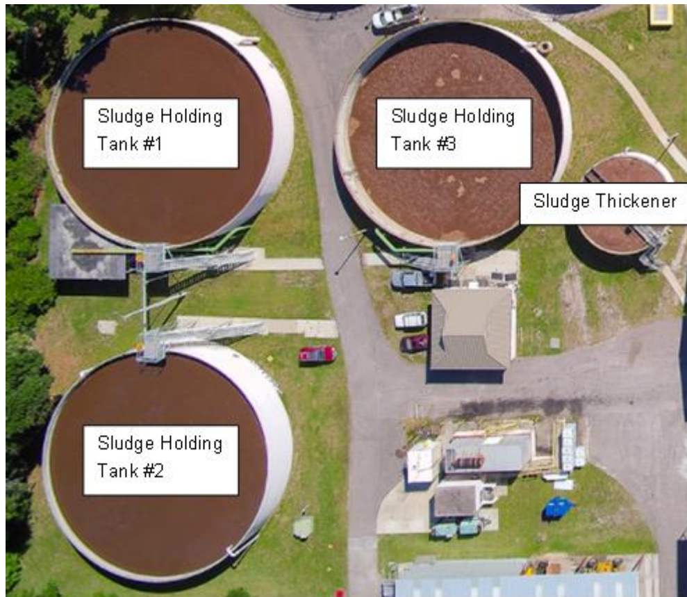
FIGURE 17: SLUDGE HOLDING TANKS AND THICKENERS
