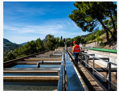
WATER AND WASTEWATER TREATMENT PLANTS
