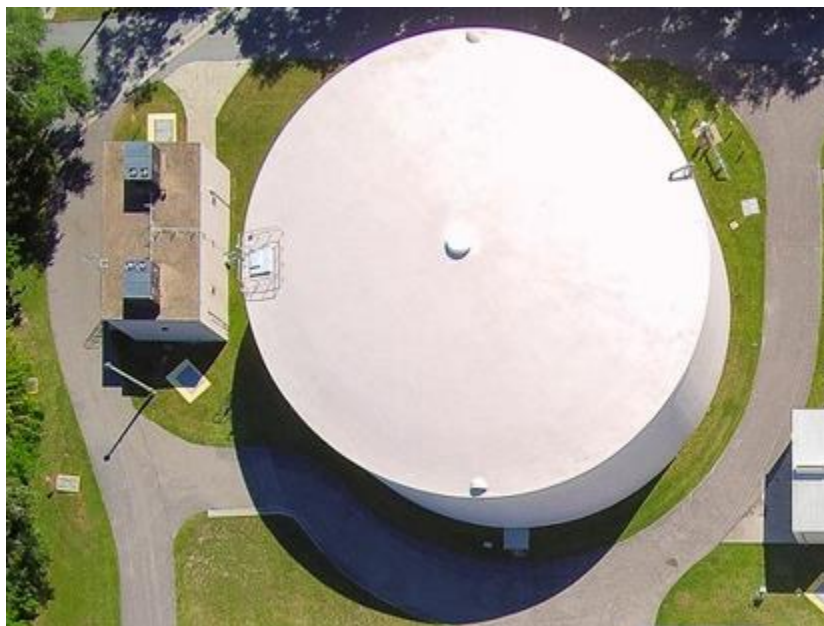
FIGURE 19: HIGH SERVICE PUMP STATION AND STORAGE TANK
