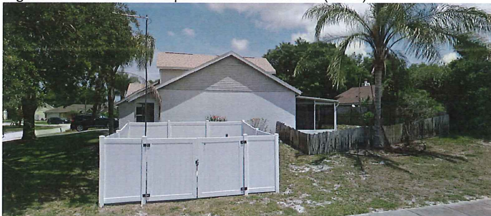
Figure 2. Lift station and previous 4-foot fence (2014)
