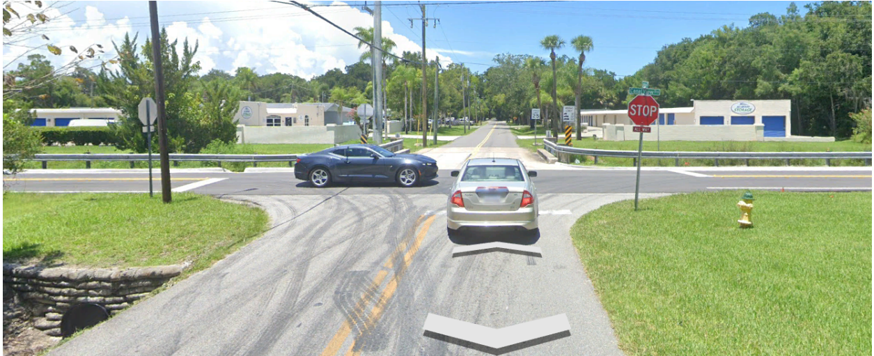
Northbound street view of bridge
