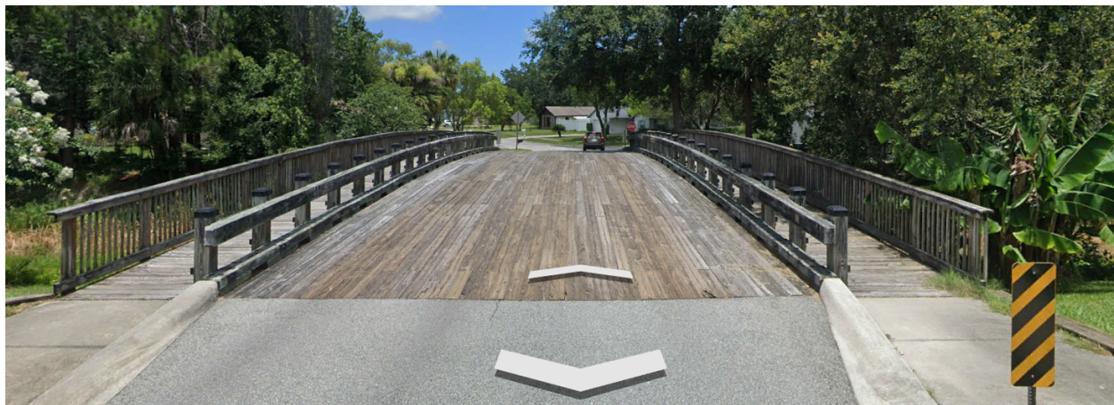
Eastbound street view of bridge
