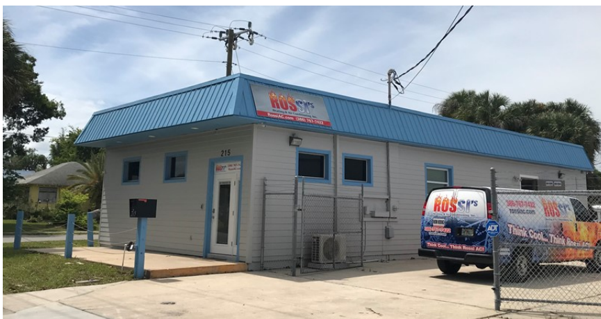
Rossi's Heat &amp; Air Conditioning – 215 Church St.
