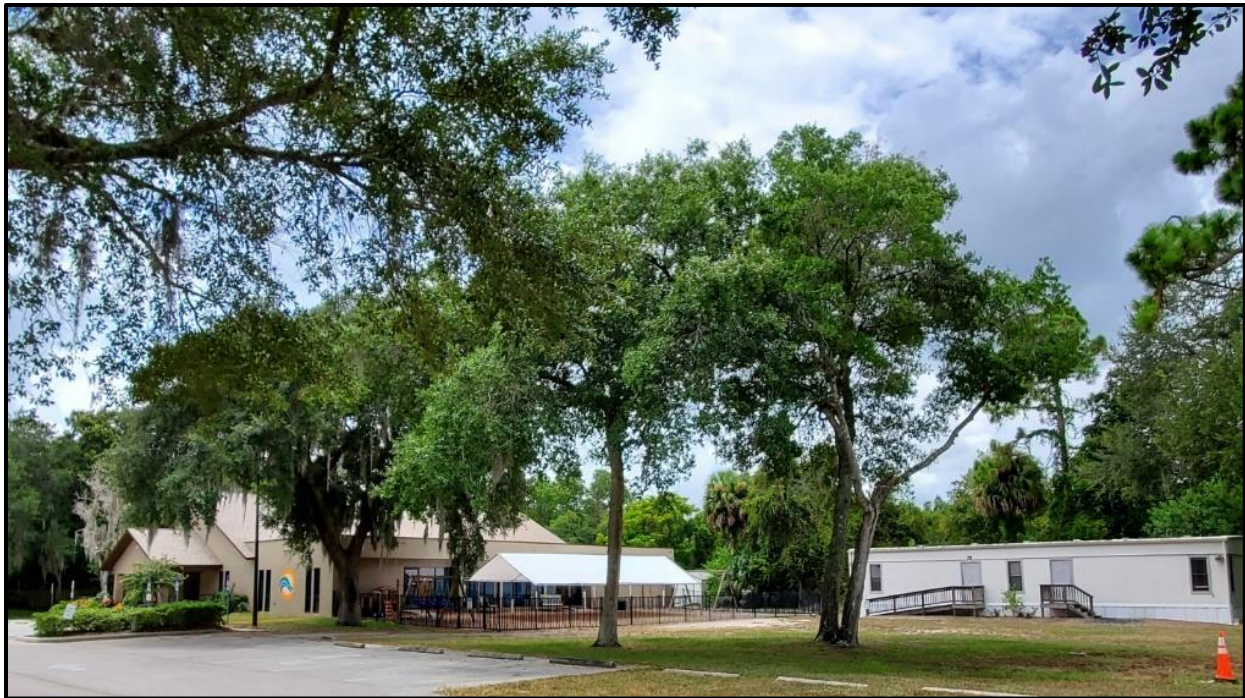
Figure 1: Existing Church and Modular Building on Subject Property
