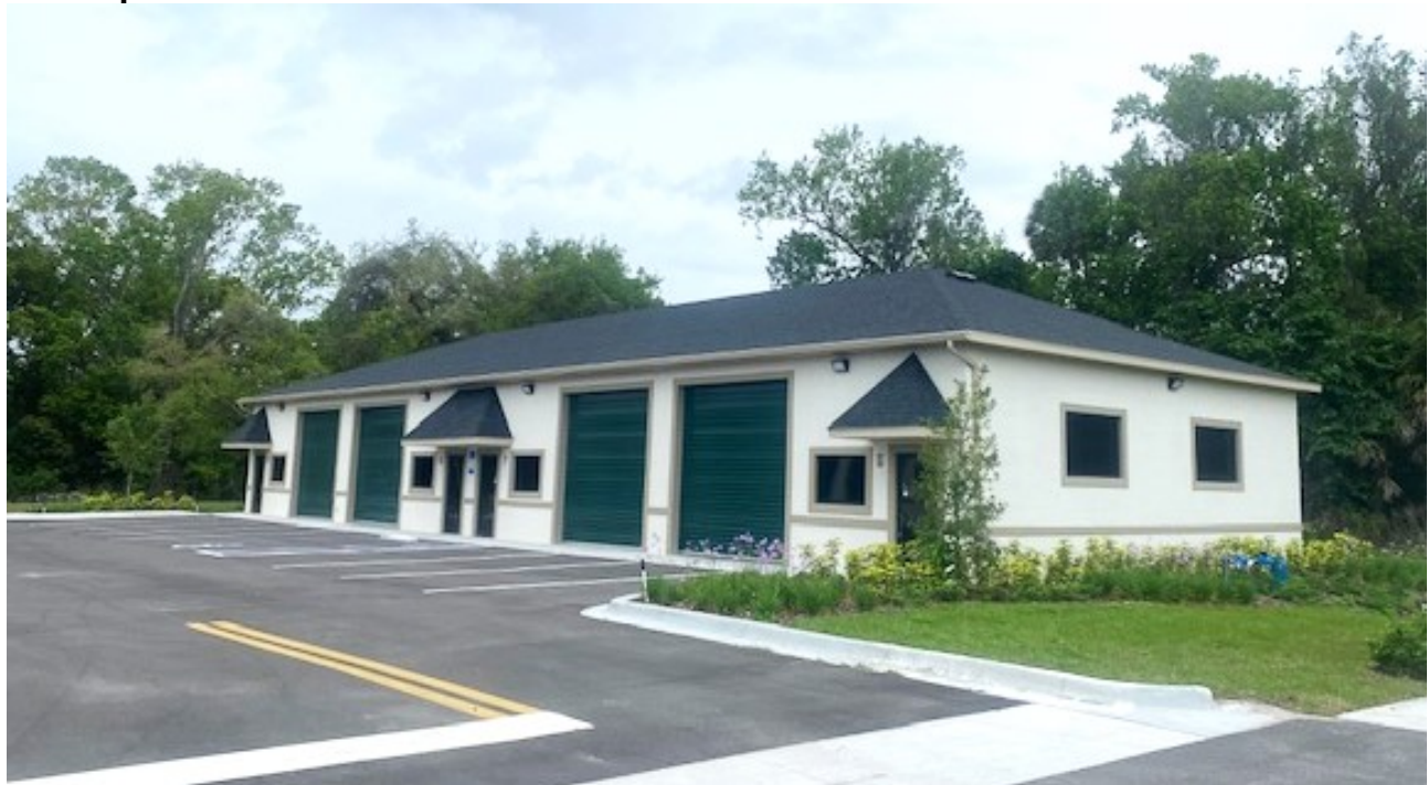
Figure 3. Typical building in the applicant's existing mini-warehouse/office facility development
