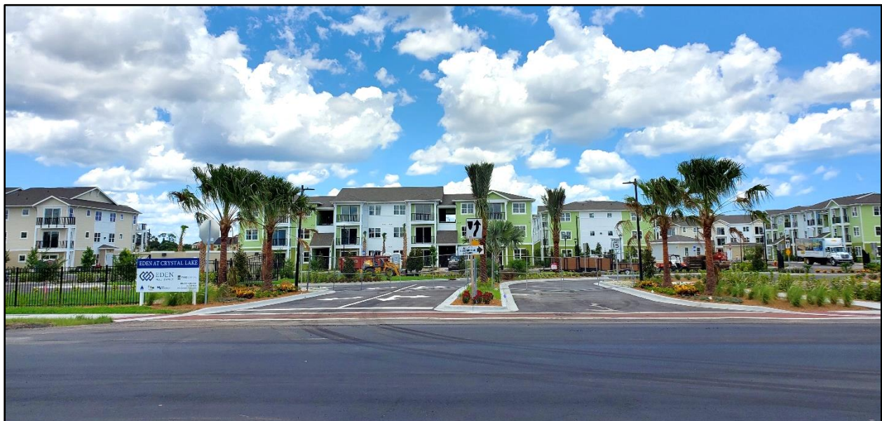
Figure 5. Entrance to Eden at Crystal Lake Apartments (Under Construction)
