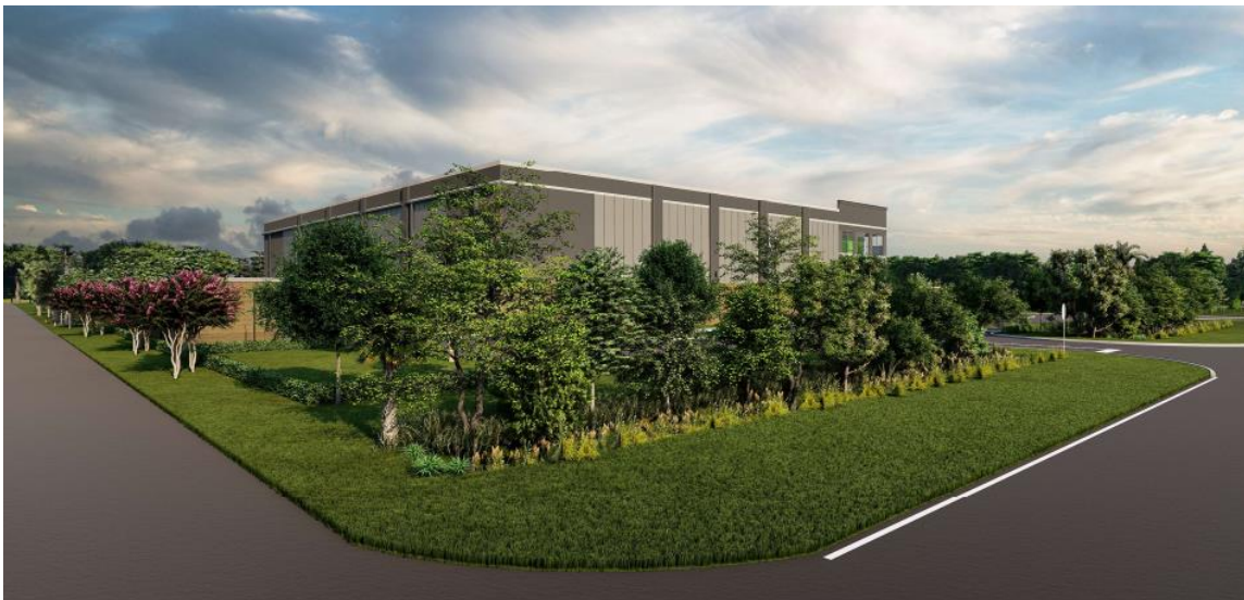
View of the elevation of the storage facility building facing the corner of Madeline Avenue and Jackson Street from the northeast corner of the site.
