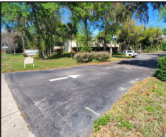
Above: Southern Driveway Entrance to Subject Property Looking Northeast
