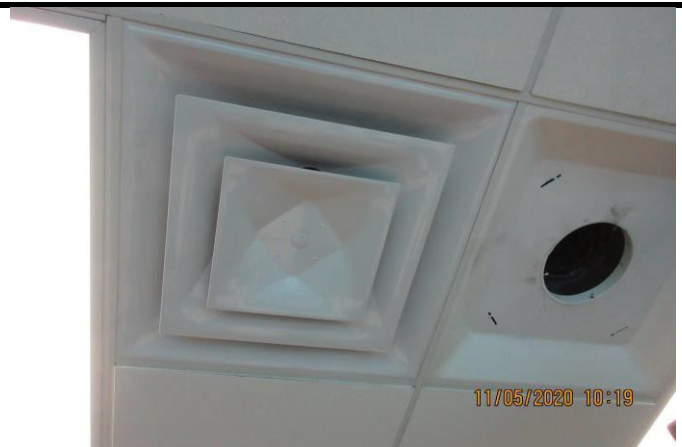
Photograph 42 Captain Fisher's Office - HVAC Duct
