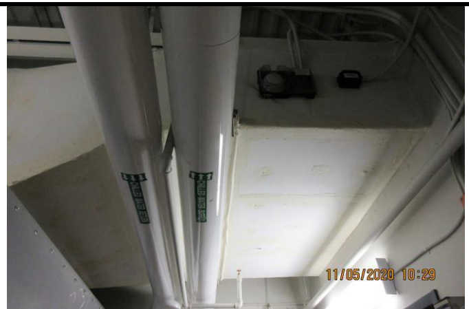
Photograph 54 Room 252 Mechanical - Plenum
