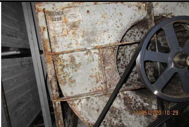
Photograph 57 Room 252 Mechanical Blower Wheel Cleaned in January 2020
