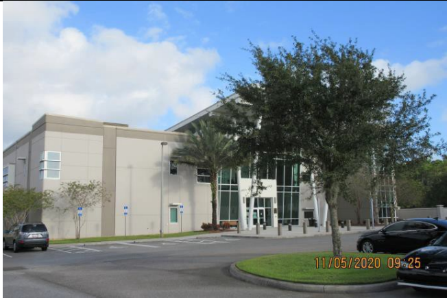
Photograph 1 Front of Building
