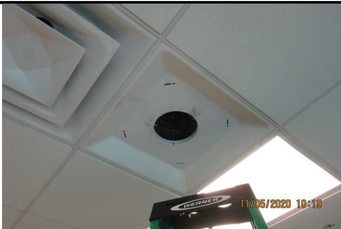
Photograph 41 Captain Fisher's Office - HVAC Duct
