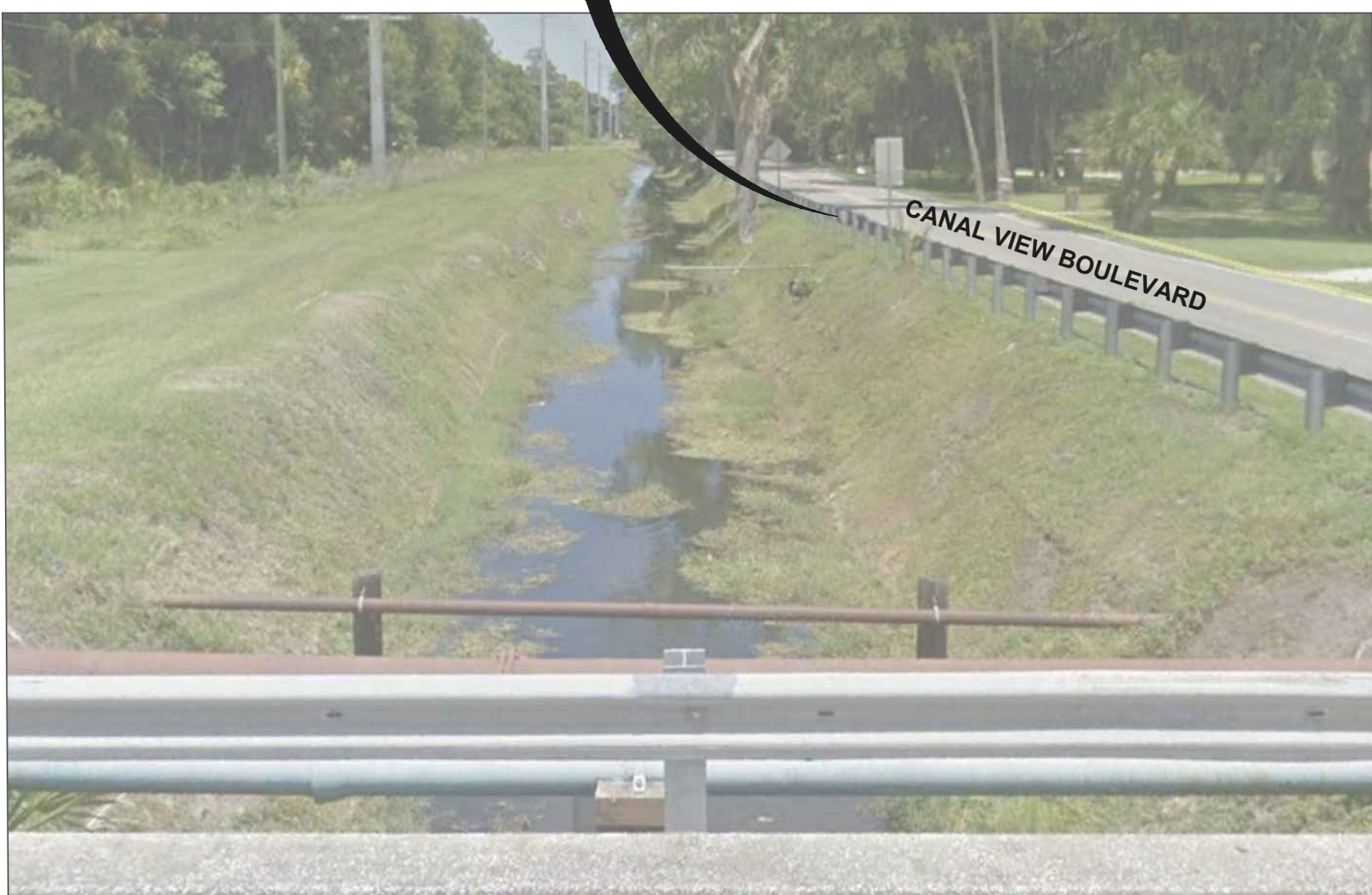
WORK AREA (LOOKING EAST FROM NOVA ROAD), NTS
