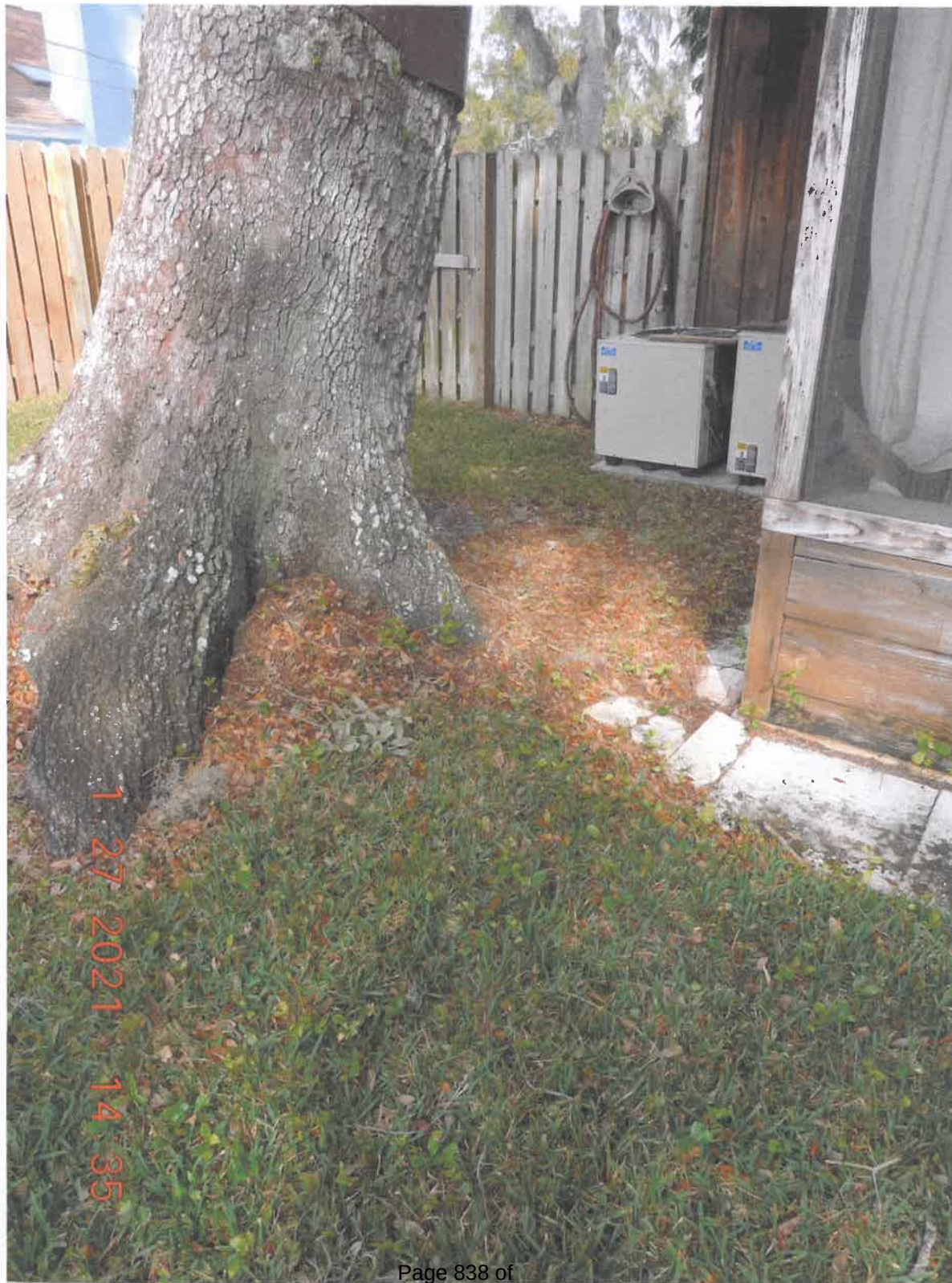
Photo of opposite viewing angle of tree trunk proximity to enclosed porch
