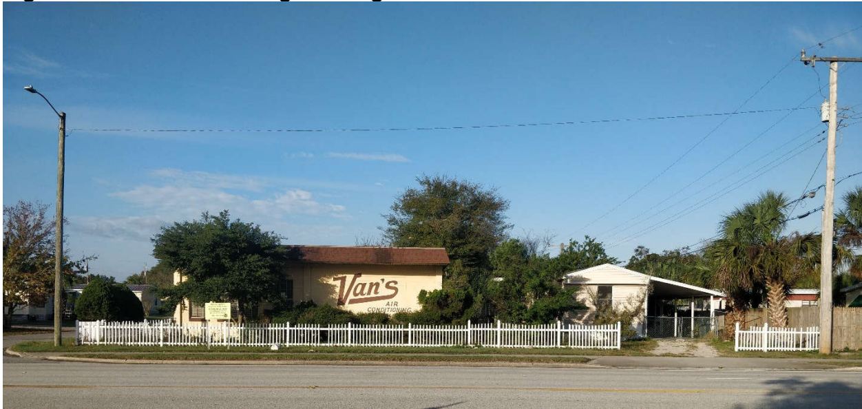
Figure 2. Picture of existing buildings
