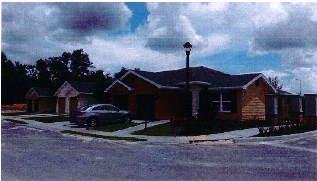
Vista Park, Hernando County, FL Under Construction
