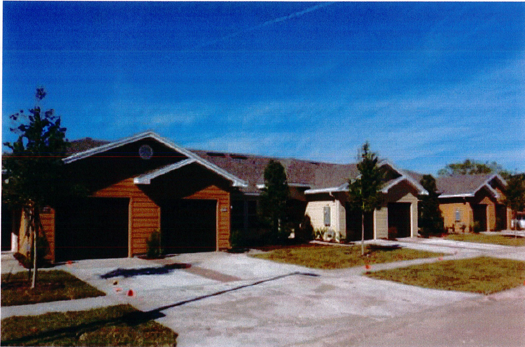
Boca Palms, Kissimmee, FL Under Construction
