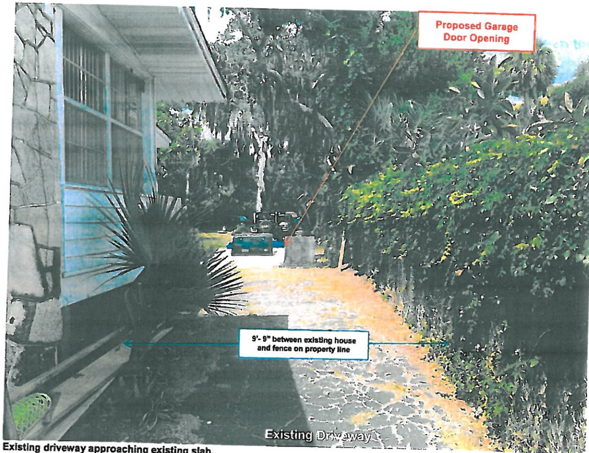
Existing driveway approaching existing slab.
