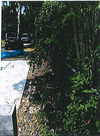
Slab of previous garage
