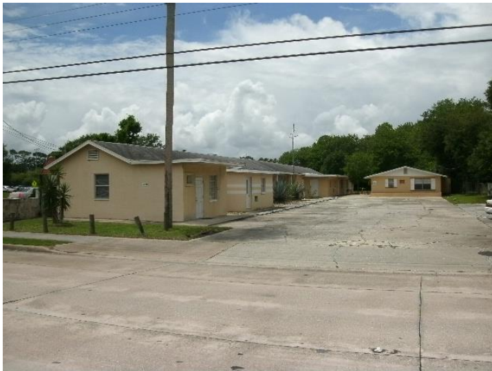
View of subject looking westerly from Ridgewood Avenue
