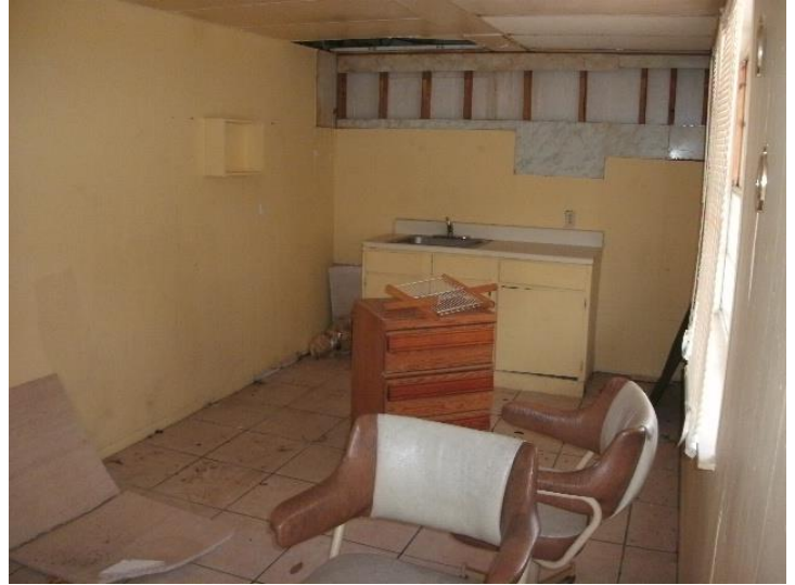
Typical interior view of subject Unit #7
