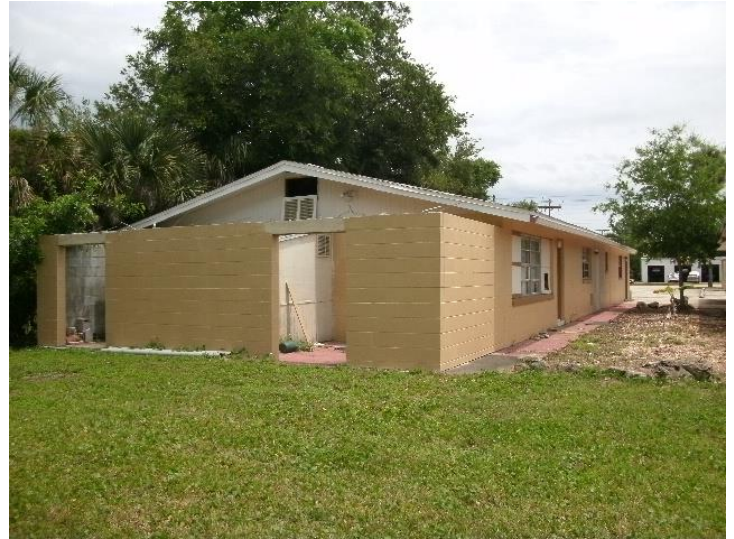
Rear view of the northerly subject building looking southeasterly
