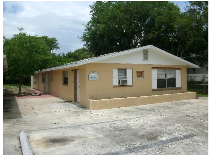
View of the northerly subject building looking southwesterly
