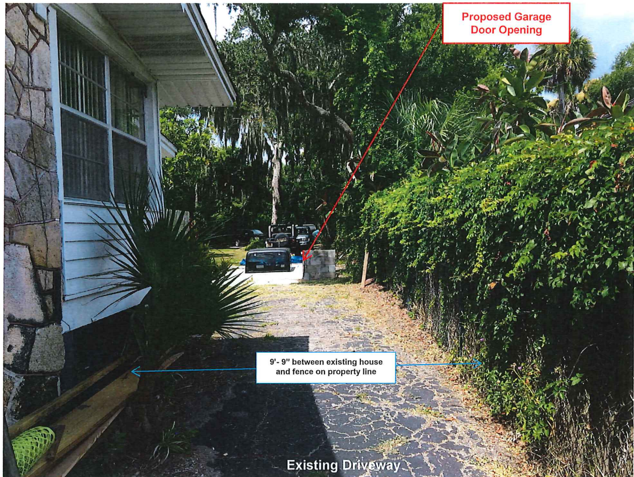
Existing driveway approaching existing slab.
