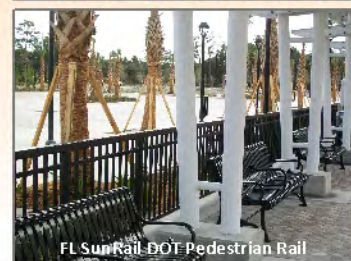
FL SunRail DOT Pedestrian Rail
