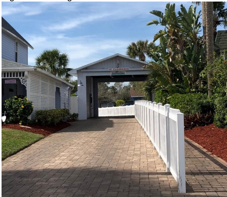
Figure 3. Existing entrance feature structure
