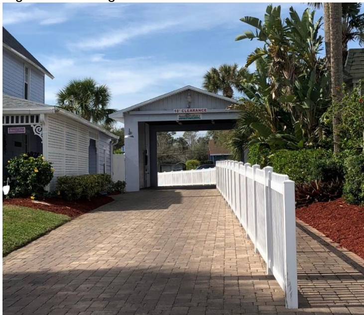
Figure 3. Existing entrance feature structure
