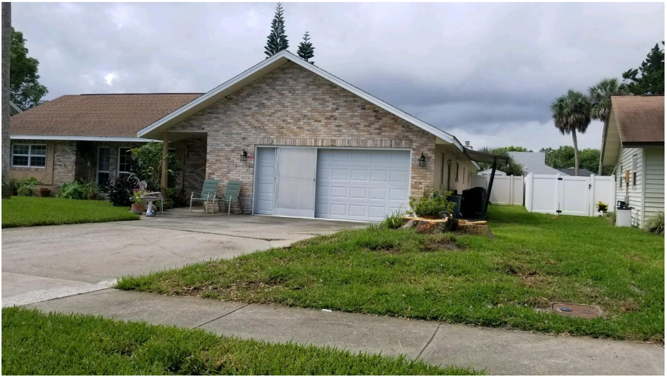
Figure 2 VIEW SHOWING STUMP AND ABSENCE OF TREES ON THE NORTH SIDE OF DRIVEWAY.
