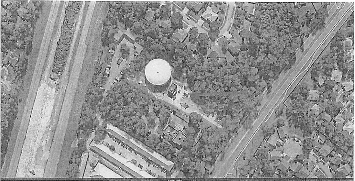
Williamson Master Lift Station - 5955 S. Williamson Blvd., Port Orange, FL 32129
